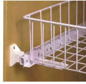
Plastic spacers are neat and uniform. These ¾-in. spacers move the side of the drawer in a little so that it won't clip the edge of the open door.
